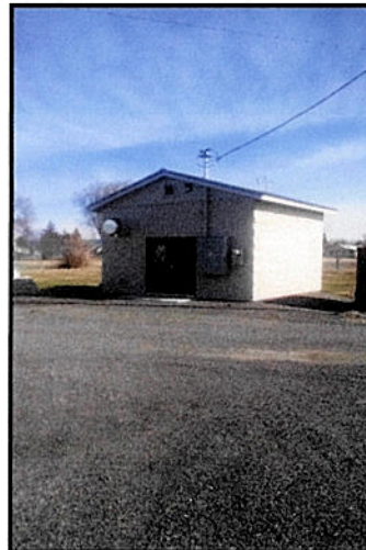
CITY OF TULELAKE BOOSTER STATION
